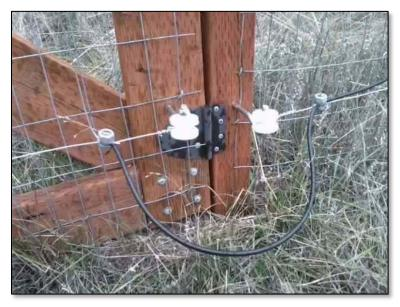
*Figure 5. Black-colored insulated electric fence wire, 12-gauge. Used here to connect the electrified lines of a gate to the main electrified lines on the fence.*
